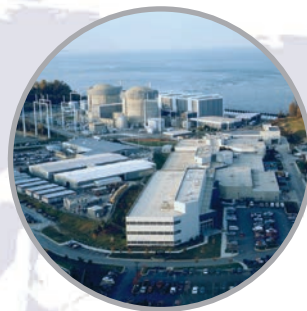
Medupi Power Station Ellisras, South Africa
